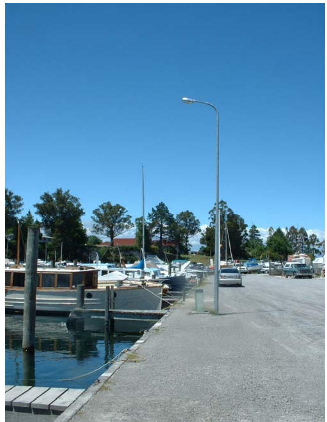
Reserve Breastwork/Mooring Lighting
