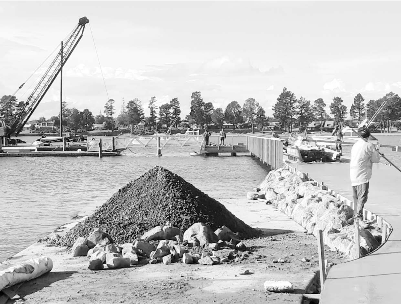
Tairua Wharf project. Thames-Coromandel District Council.
