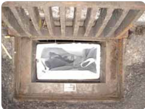
Enviropods installed in stormwater drains to filter out leaves and rubbish
