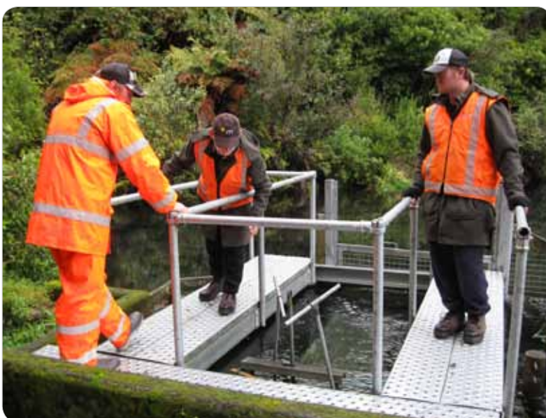
Infrastructure water team inspecting the Tirohanga water intake
