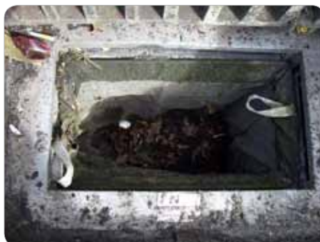
Enviropods installed in stormwater drains to filter out leaves and rubbish
