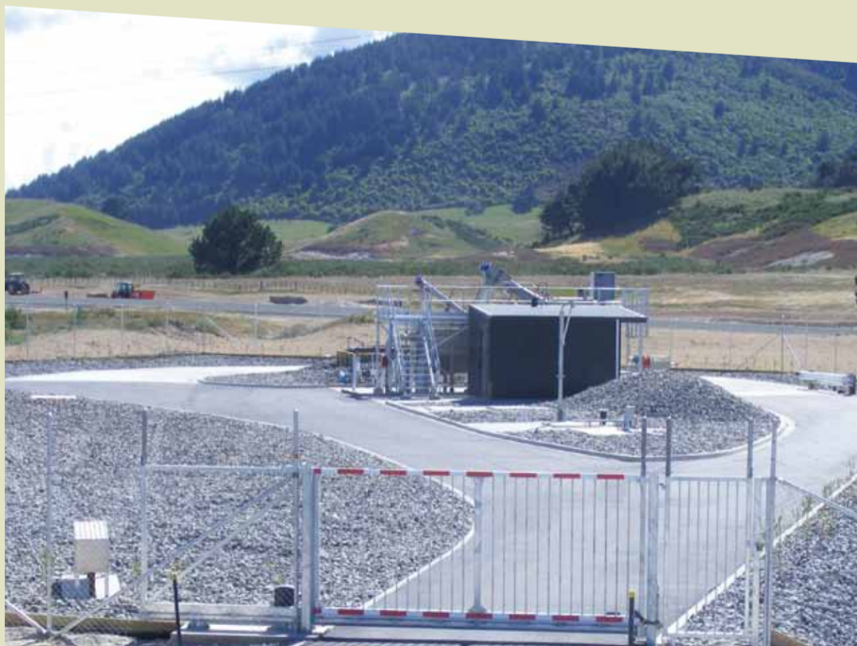
Ashwood septage reception facility
