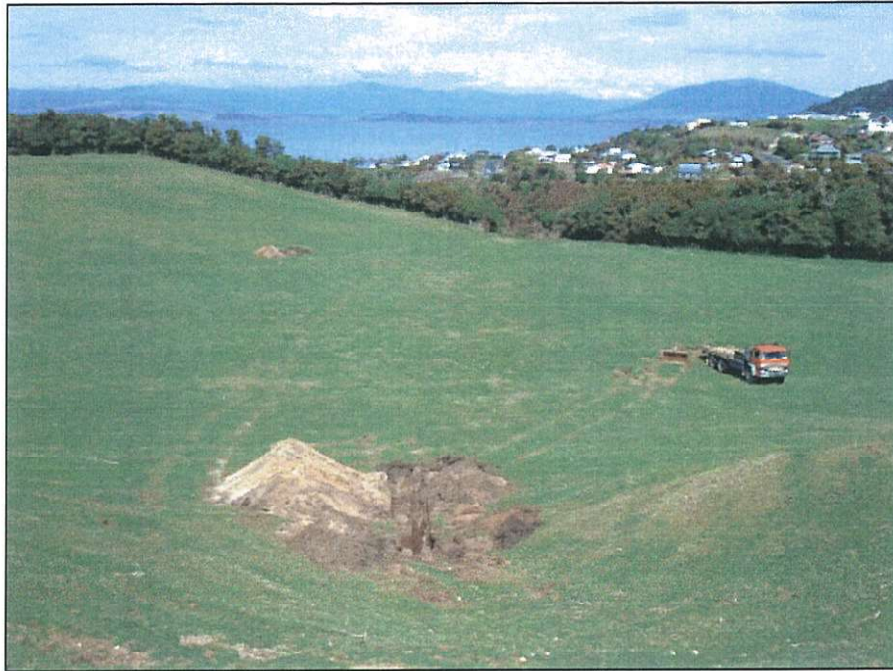
Fig. 1: View south towards the low-lying area with Lake Taupo in the distance. Test Pit No. 1 is in the foreground.
