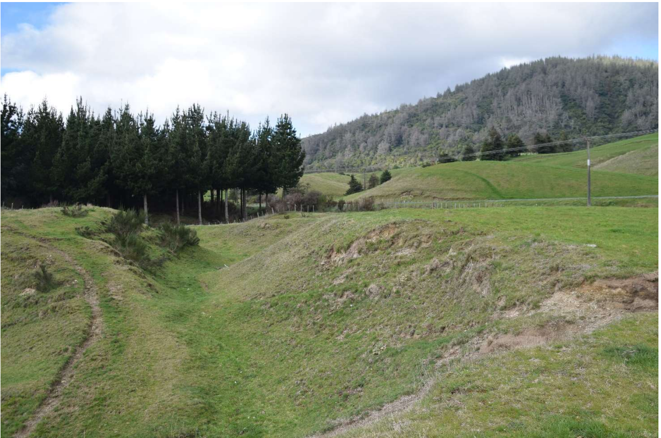
Figure 3: Example of localised instability due to erosional issues
