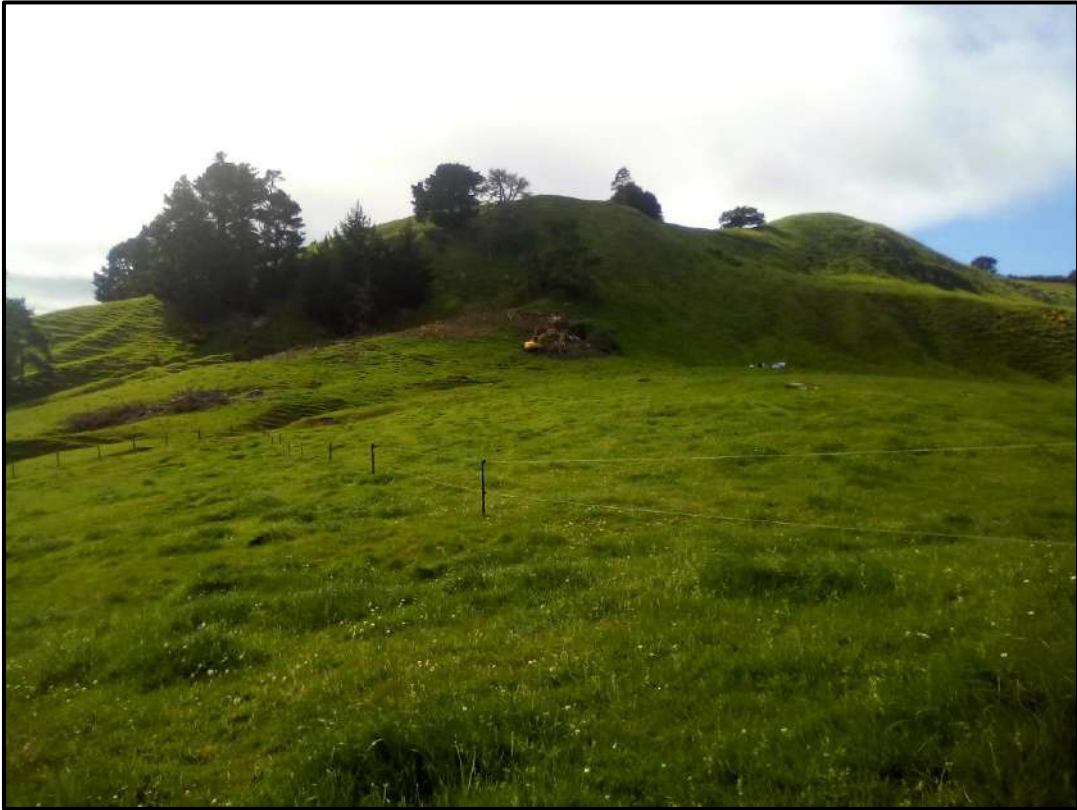
Photograph 5: Tree felling operation on the Marapa Escarpment in the northeast corner of the subdivision site.
