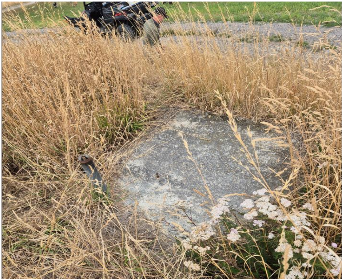
Figure 6. Concrete pad with mounting bolts inspected during the 2025 survey indicating location of water pump noted by Fletcher in 1978.
