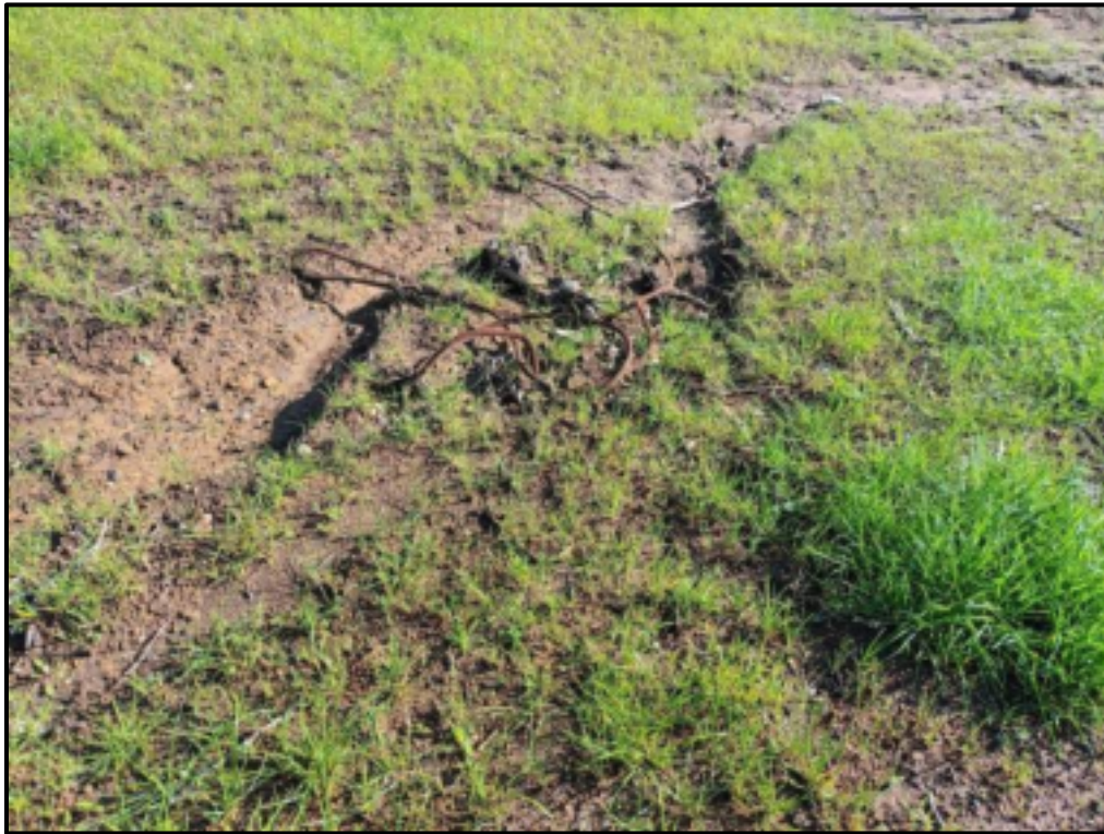
Photograph 6: Cable Remaining in the Cleared Gully in the North of the Site (24 May 2023).
