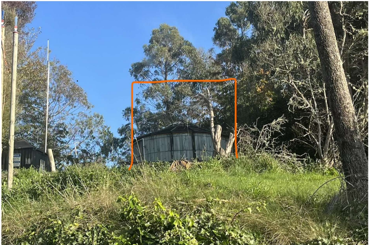
Fig. 2: Existing water reservoir at Blue Ridge Drive as viewed from the property at 72 Blue Ridge Drive, Taupō
