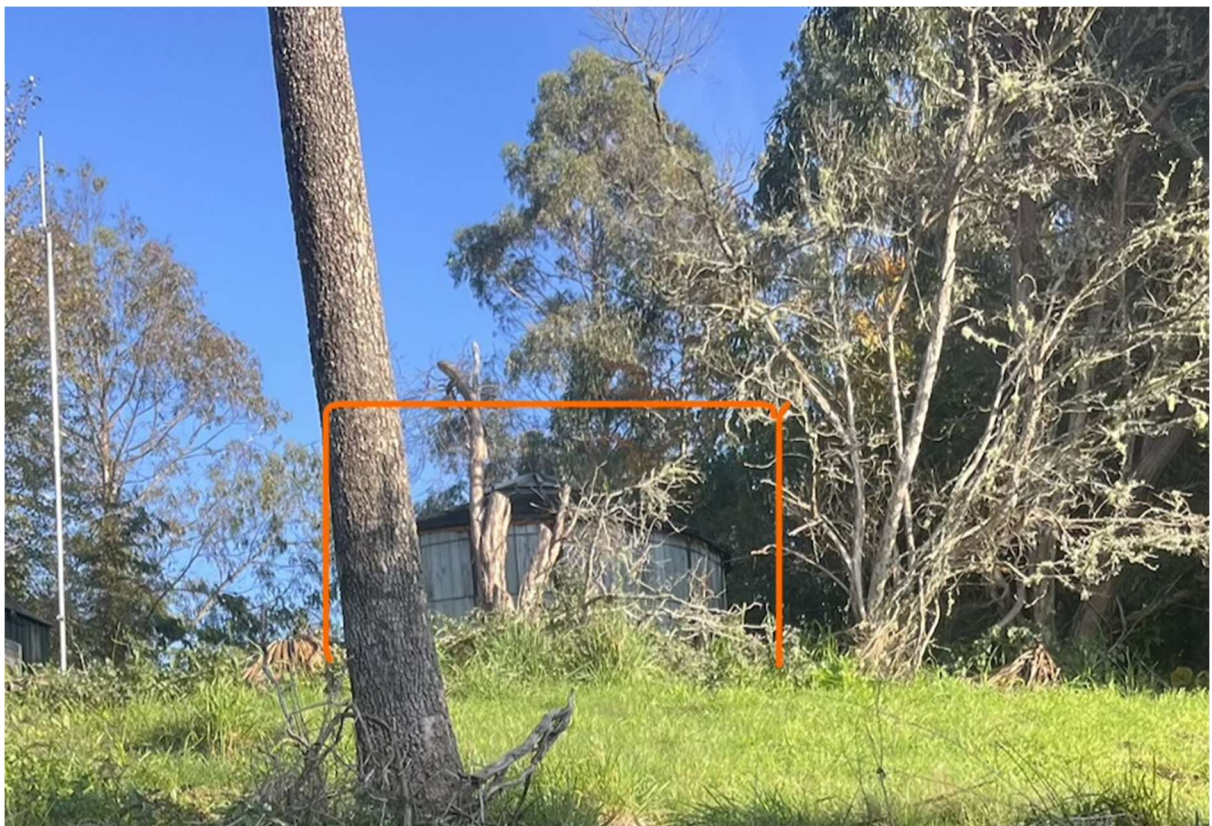
Fig. 3: Existing water reservoir at Blue Ridge Drive as viewed from the property at 72 Blue Ridge Drive, Taupō
