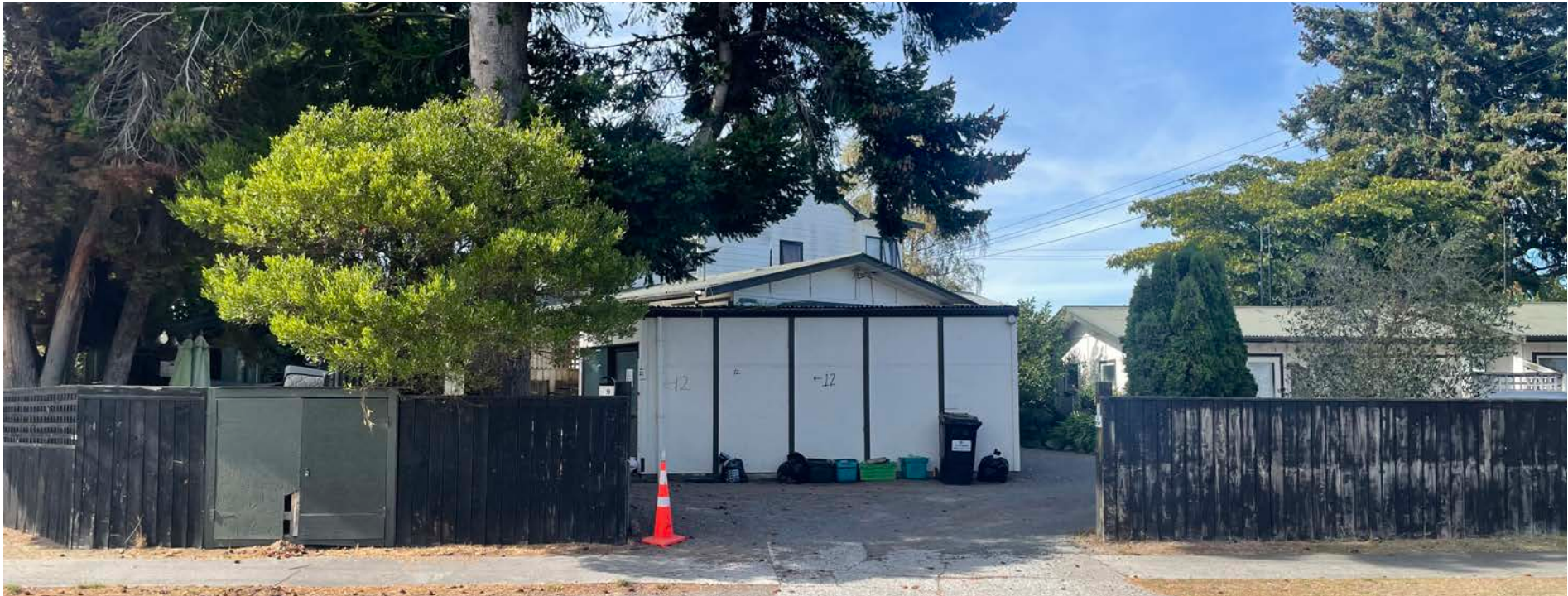
View from Charles Crescent looking towards corner of site. Existing driveway, buildings, trees and power box
