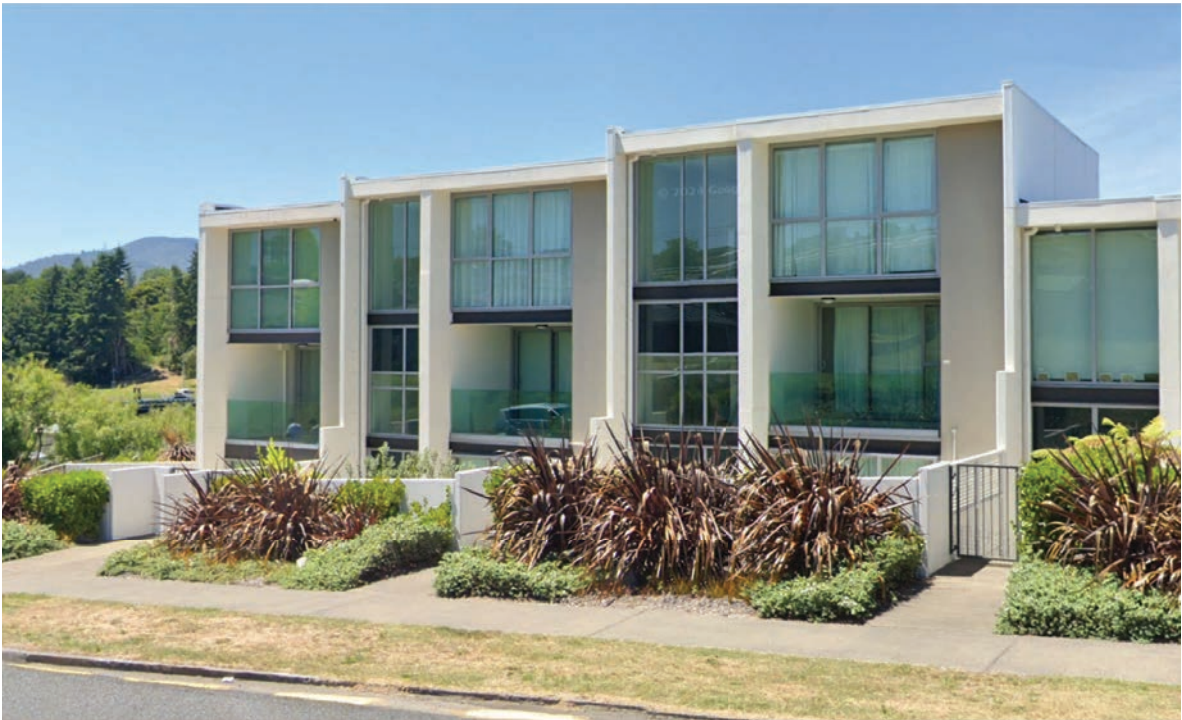
Photograph of Norman Smith Street development (view from street showing 3-storey terraces)
