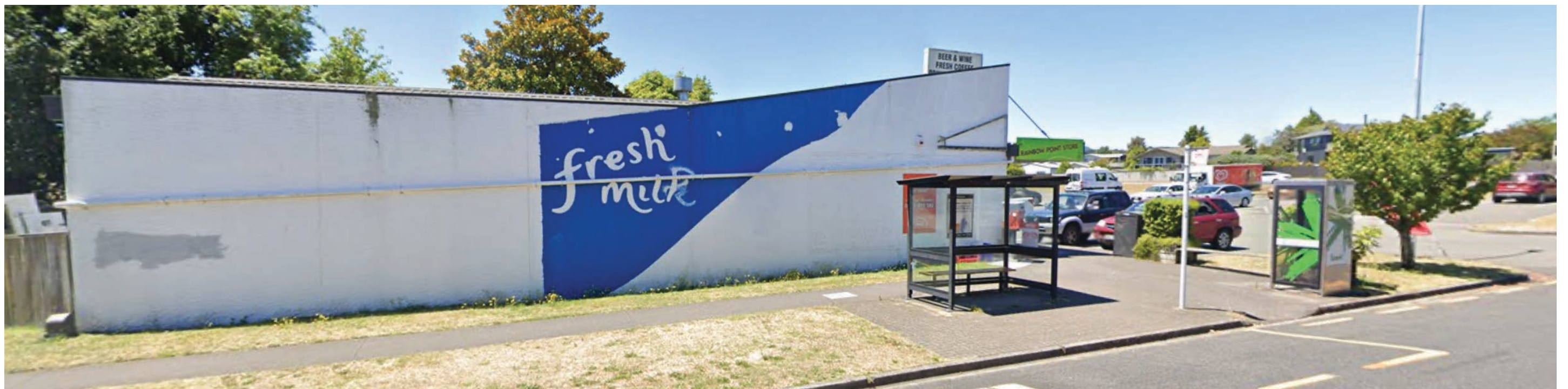
Google street view showing blank commercial facade with no set back directly opposite the site fronting Rainbow Drive
