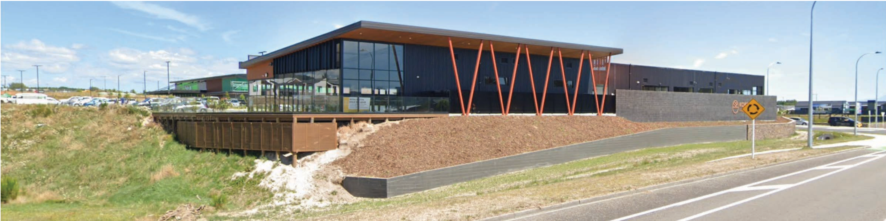
Photograph showing the Lake Terrace facade of Kokomea Village (commercial) with the supermarket in the background
