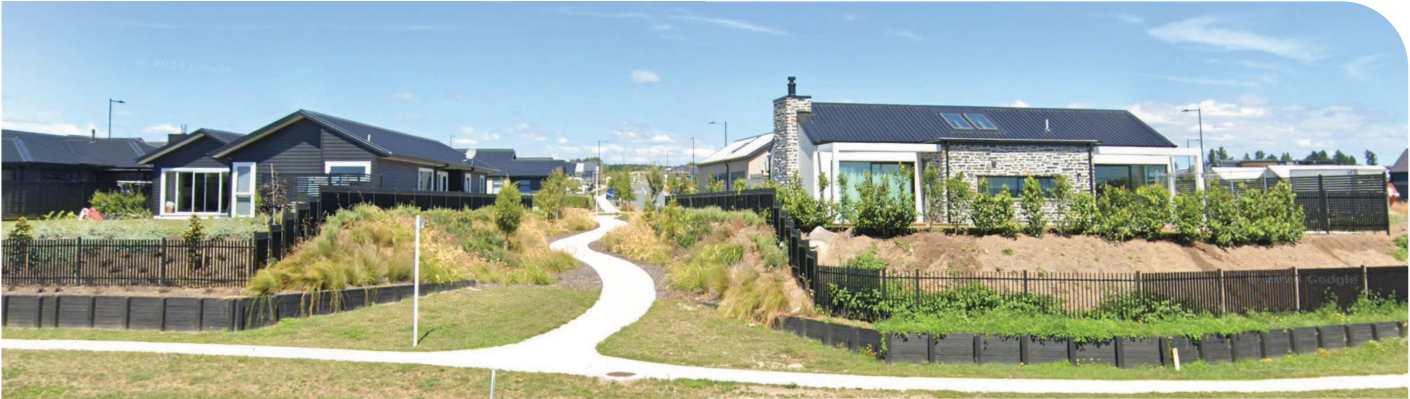
Extract from Google Street view showing single level homes elevated approximately 3m above Lake Terrace - Homes off Ngaru Terrace (opposite Rainbow Drive)
