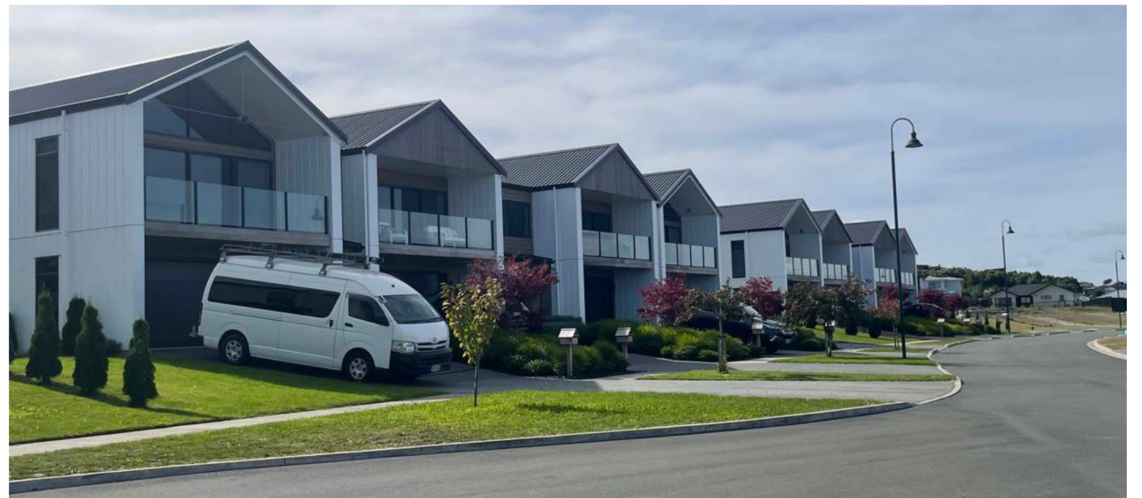
Photograph showing 2-storey townhouse development at Blue Dun Place
