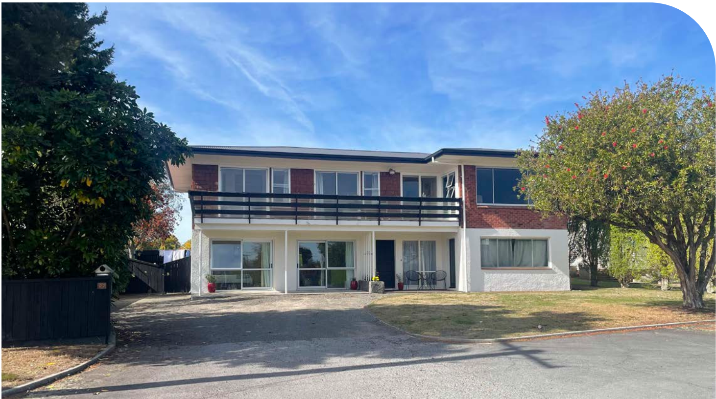
Photograph showing 2-storey home at 25 Charles Crescent (immediately adjacent to site)
