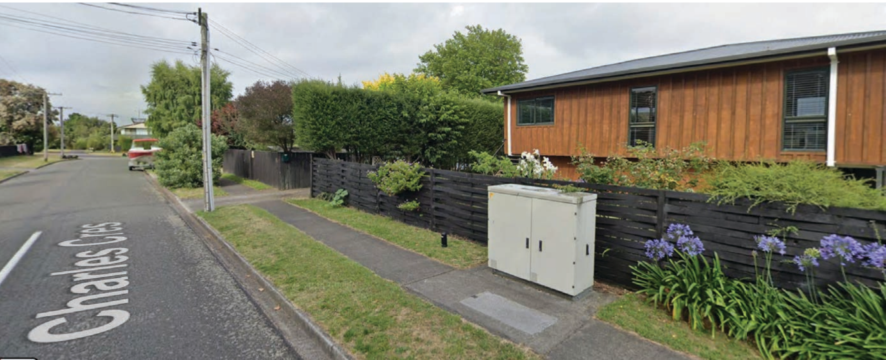
Google street view showing opposite side of Charles Crescent (2-storey home on corner of Charles Crescent and Rainbow Drive)
