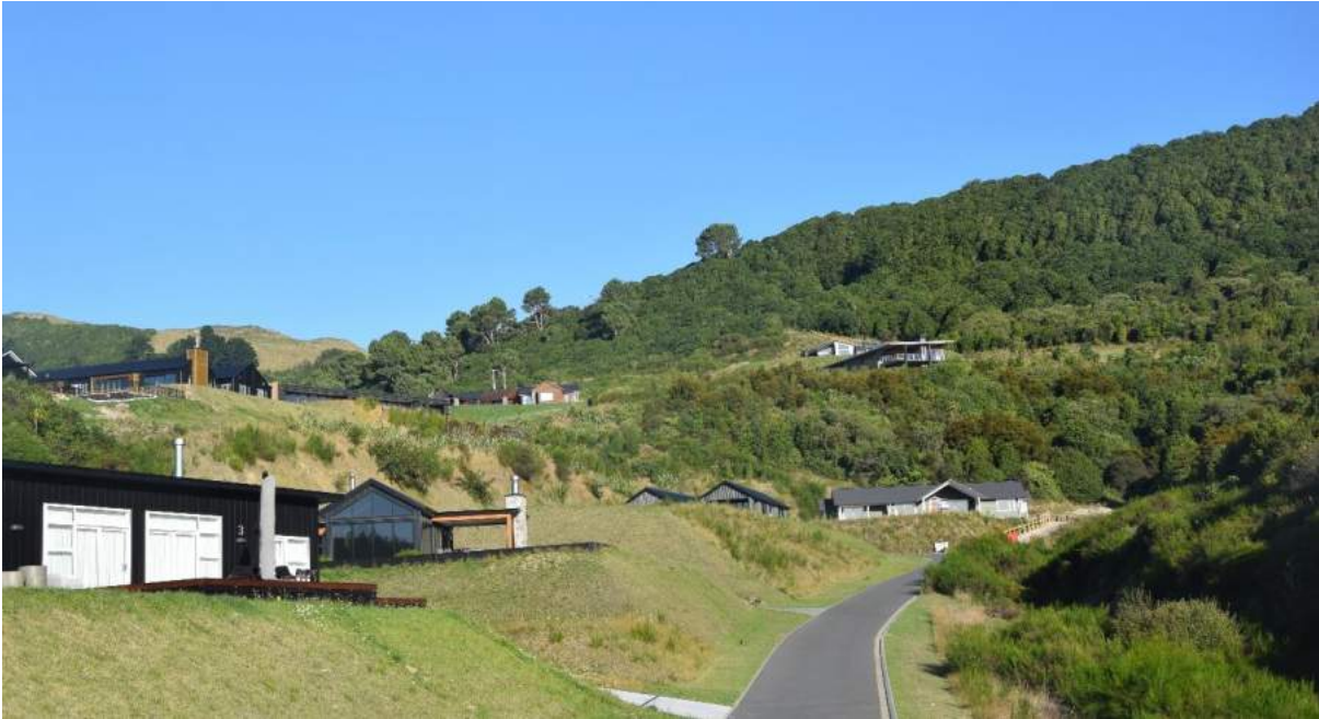
Figure 18 Example of earthworks for building platforms undertaken within the localised area.
