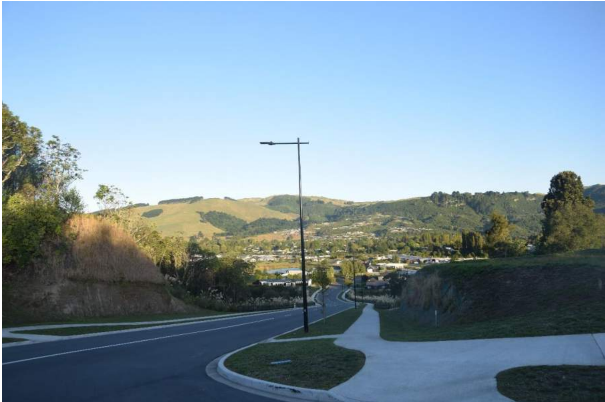
Figure 12 New roading for expanding residential development within Kinloch.
