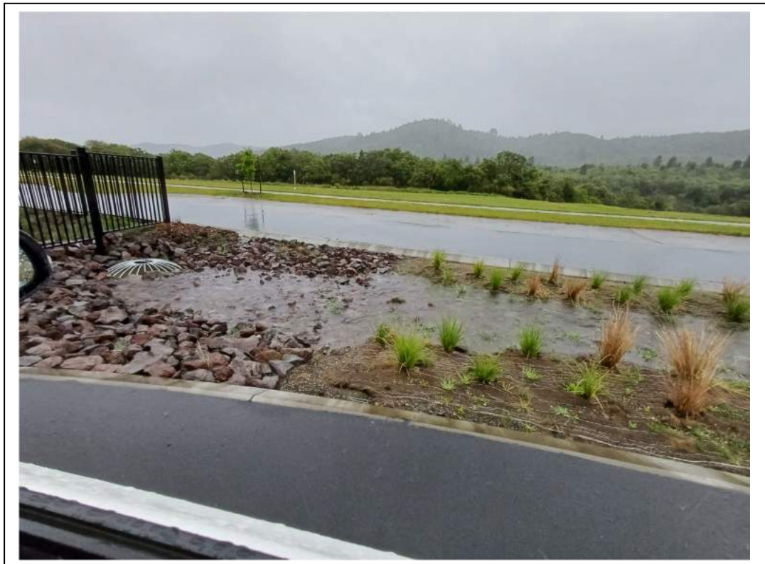
Photo 2 – Swale Inlet to Pond
