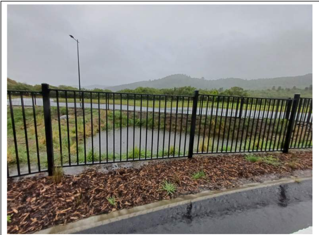
Photo 6 – Stormwater Pond Forebay
