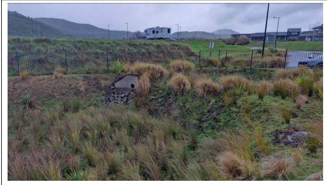
Photo 13 – Vegetated Attenuation Pond Sample – May 2025
