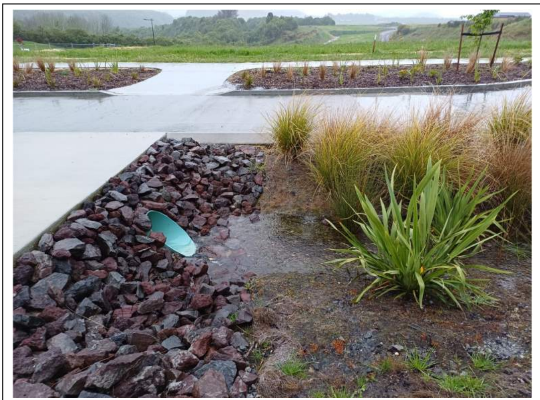
Photo 3 – Swale Under Footpath (Inlet)
