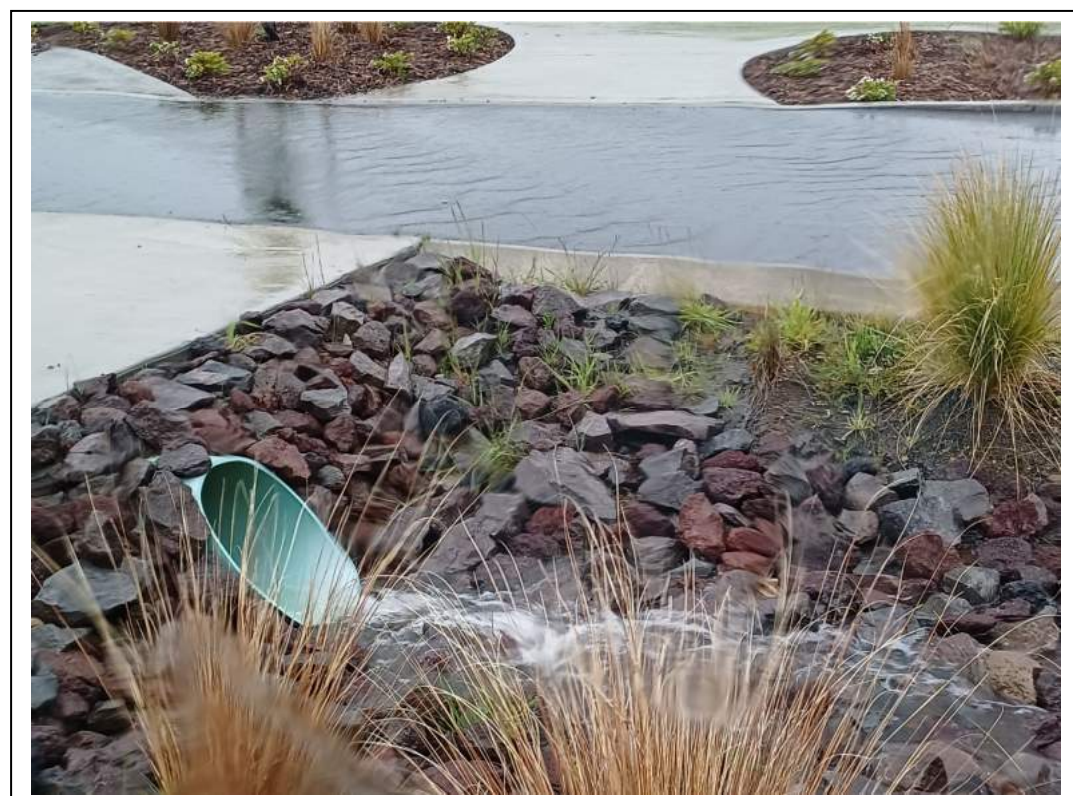
Photo 4 – Swale Under Footpath (Outlet)
