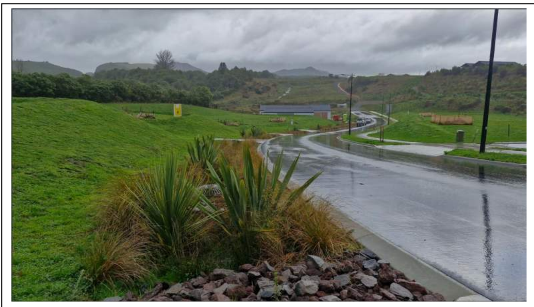
Photo 8 – Vegetated Swale Sample 1 – May 2025
