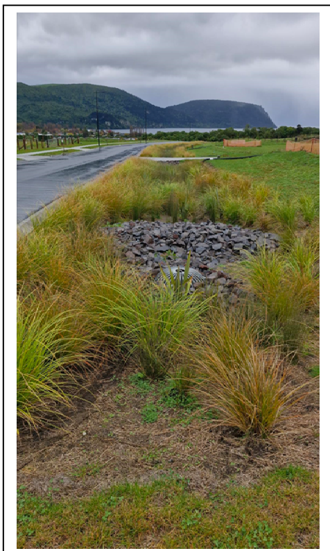
Photo 10 – Vegetated Swale Sample 3 – May 2025
