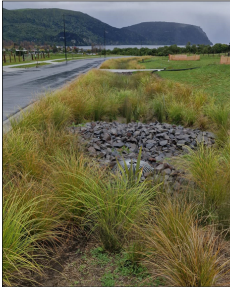
Figure 6: Vegetated Swale within Durmast Place
