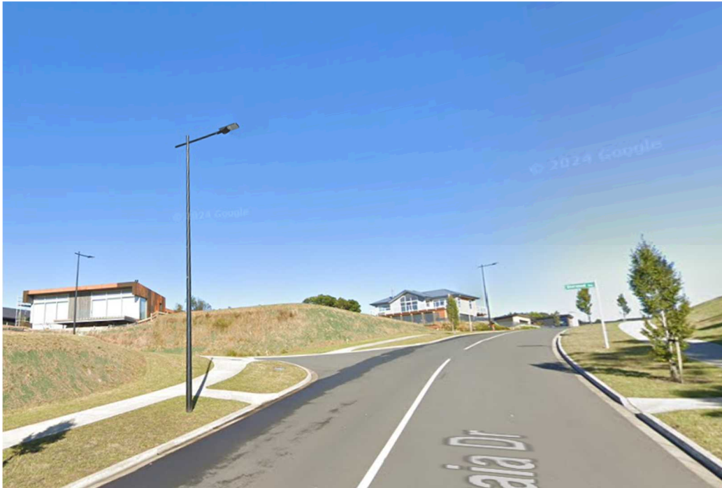
Figure 1: Image of Street lights along Okaia Drive Stage 1 Seven Oaks
