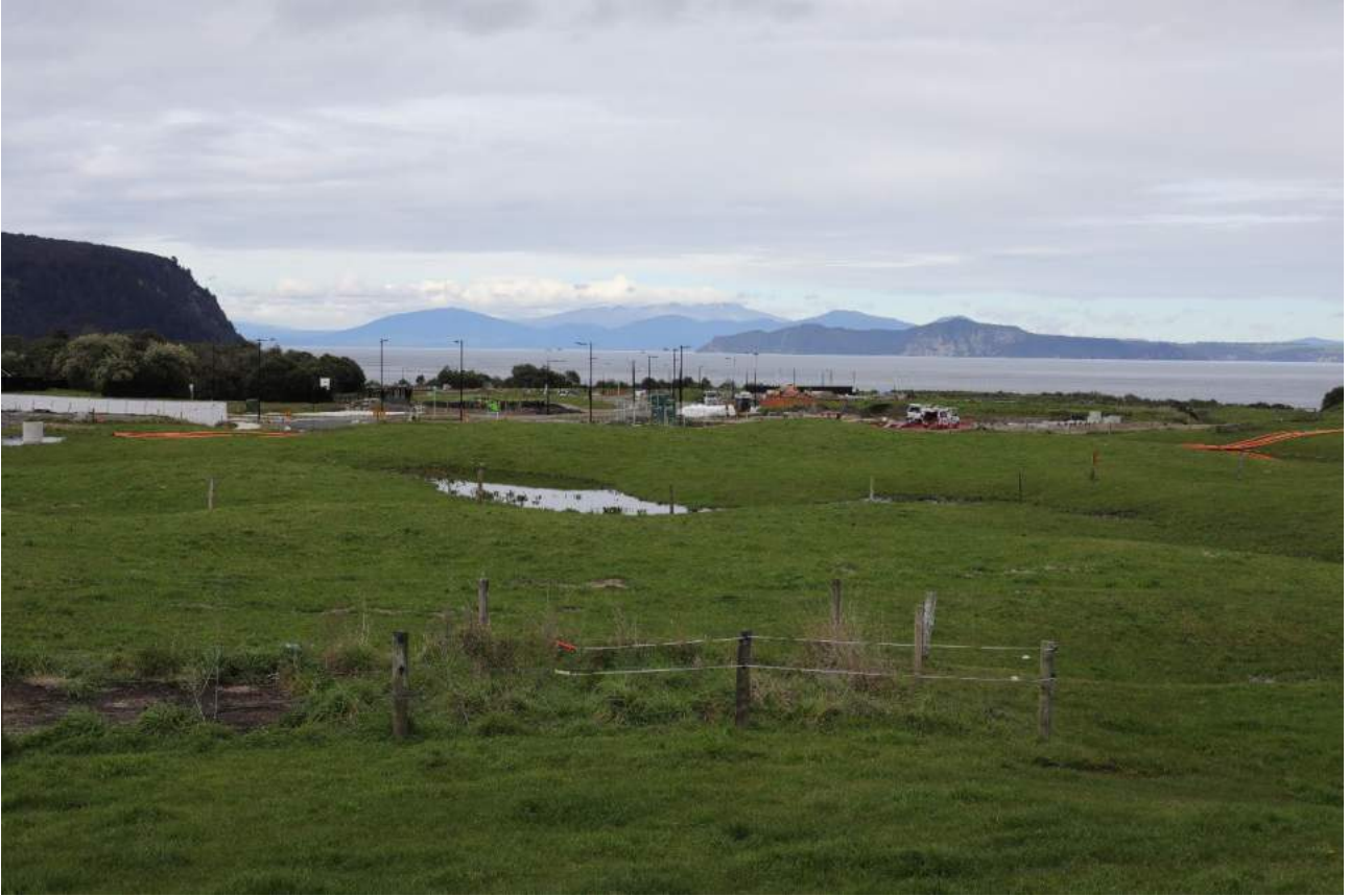
Figure 3: View from within the application site looking south to the consented subdivision under construction.
