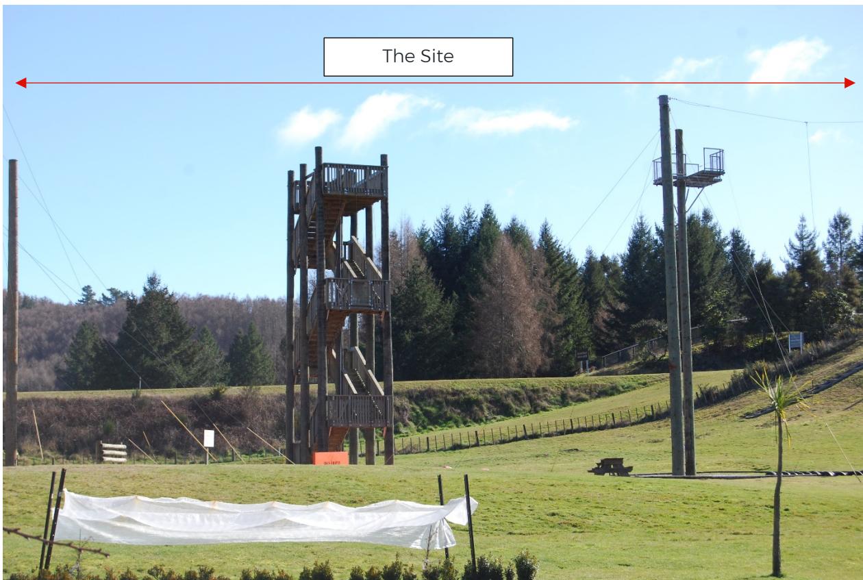
Figure 6.5 Representative view 3 looking north west from the Huka Honey Hive carpark towards the Site.
