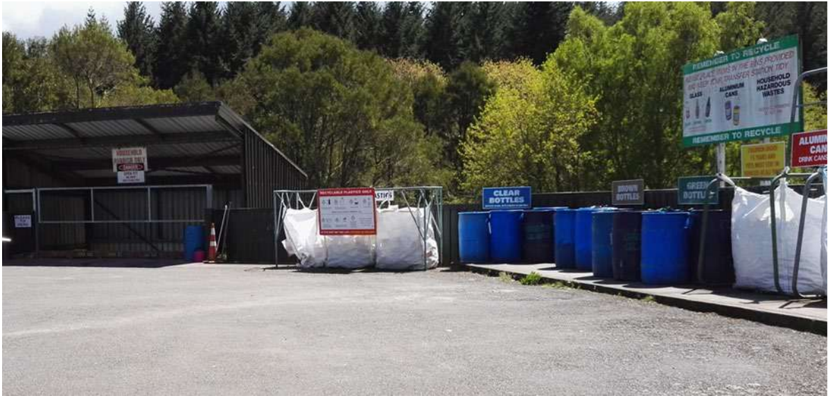
Figure 1: Broadlands Road Recycling Facility
