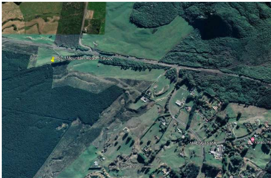
Figure 1: RNZ's radio transmission Facilities at Mountain Road, Taupō
