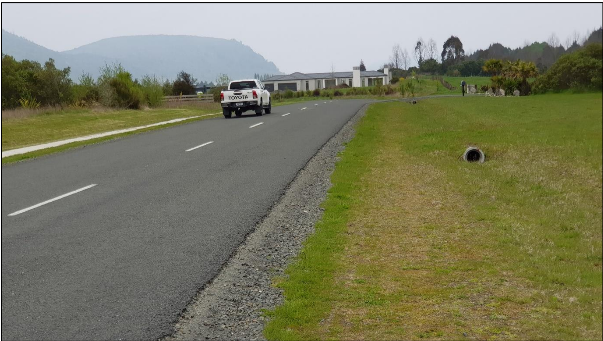
Figure 18: rural residential roads like Oakdale Drive have a rural cross section and again will be difficult to achieve operating speeds of even 50 km/h
