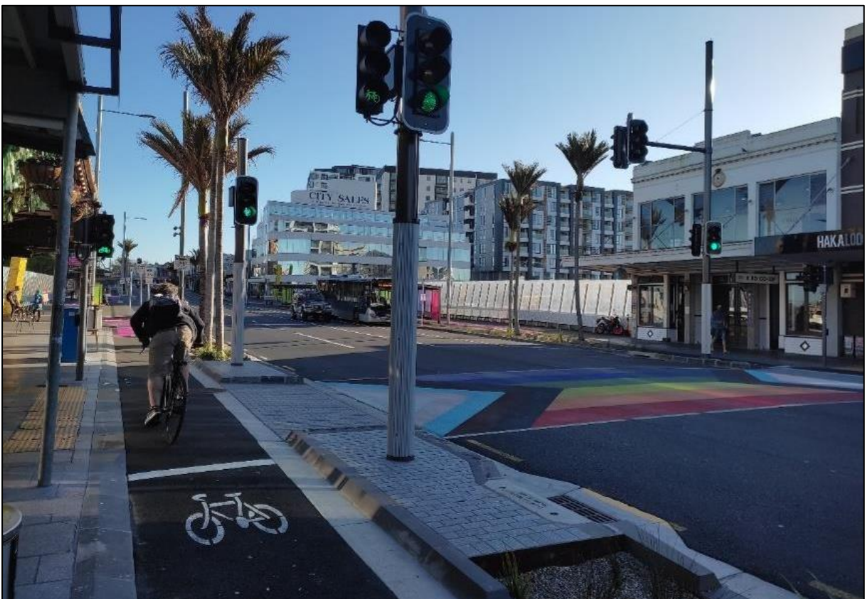
Figure 4 Separated cycle facilities
