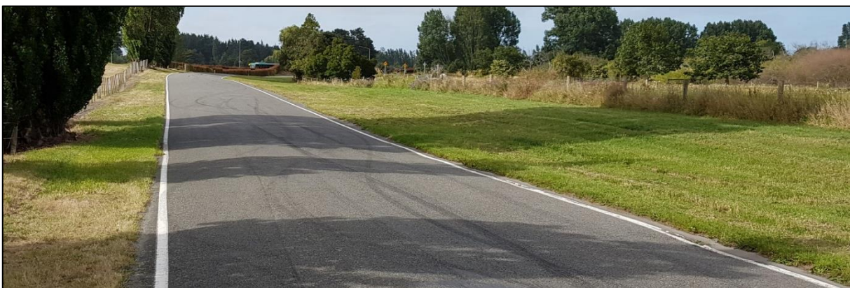
Figure 10 Removal of centreline on rural road
