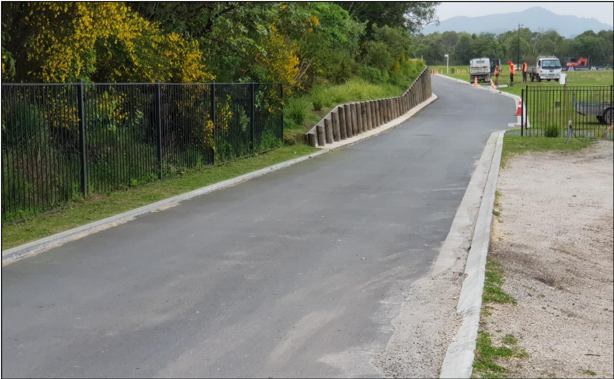
Figure 19: New short/narrow streets like Sherwood Way have tighter curves and pedestrians walking in the street, hence may have low operating speeds and be “self-explaining” at 40 km/h or less
