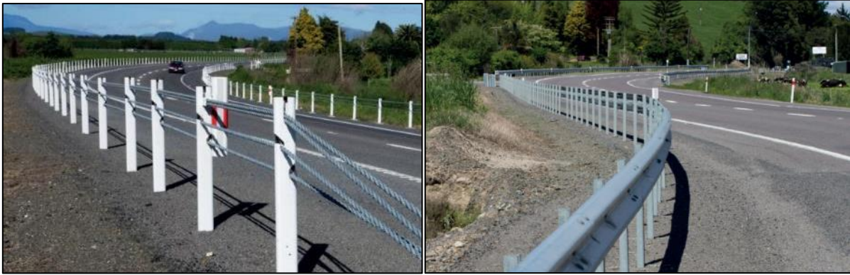
Figure 7 Flexible road safety barrier and guardrail on rural roads (Waka Kotahi)
