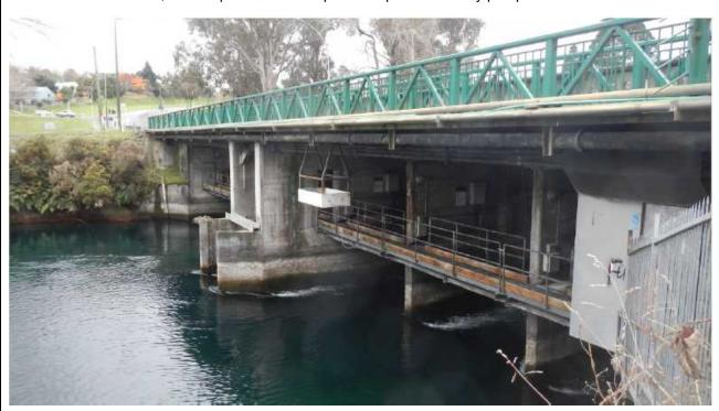
The proposed solution includes upgrade of the pipeline across the bridge from its current material and size (200mm steel), to a larger 300mm concrete lined steel pipeline. It includes upgrade of support structures and brackets as required to ensure future resilience of the pipeline. The pipeline will connect into the upgraded DN355 PE pipelines to be installed during 2021 as part of the Acacia Bay connection to Taupo project.
