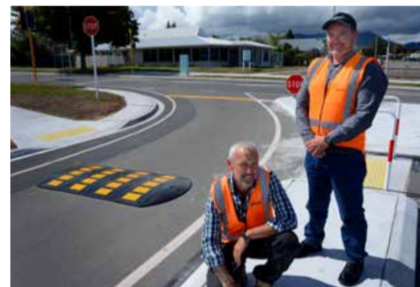
Downer crew with the new speed cushion on Horomātangi St.
