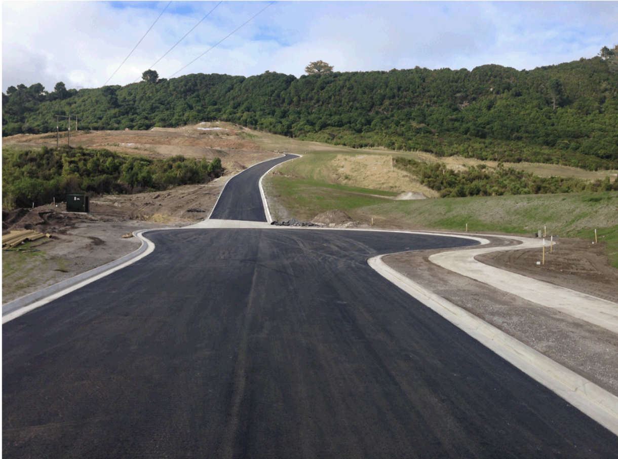
Photo: June 2014, before houses & entrance gate. This was Stage 3 of Locheagles.
