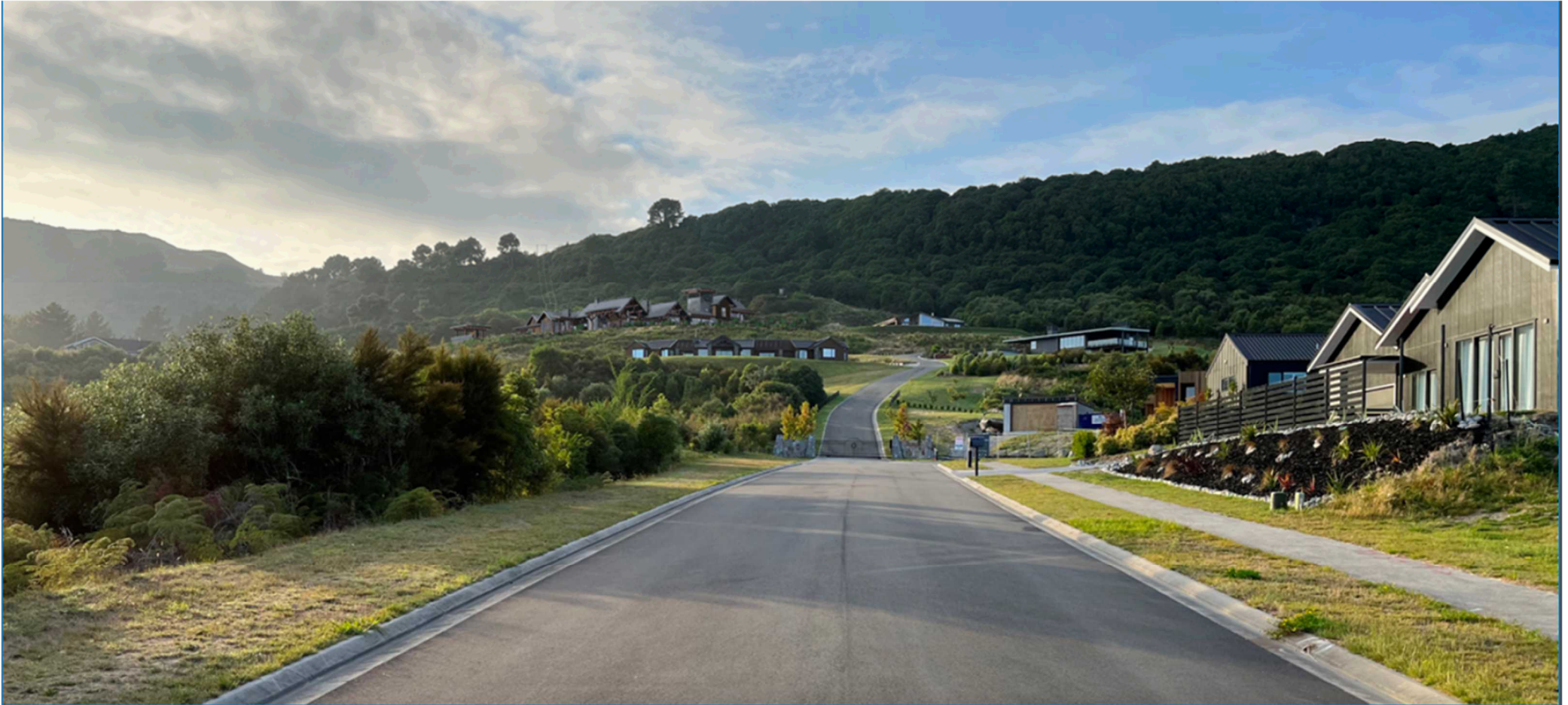
Visual Simulation - Top of Locheagles Rise, 9 March 2022. The vegetation surrounding the house is estimated at 5 years growth
