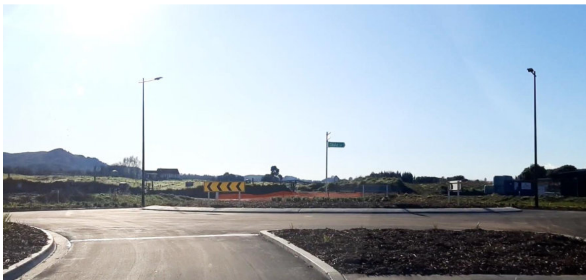
Figure 7: Okaia Drive / Kahikatea Drive roundabout intersection (Okaia Drive left to right, Kahikatea Drive straight through)
