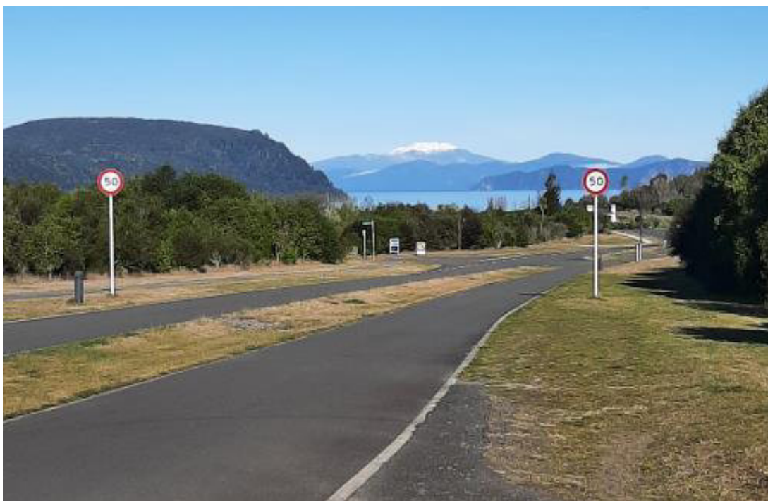
Figure 14: Oakdale Drive northern end - at the intersection with Whangamata Road
