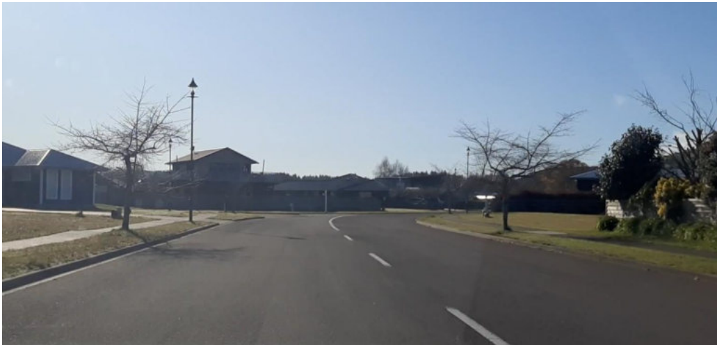
Figure 18: Lisland Drive north of Okaia Drive
