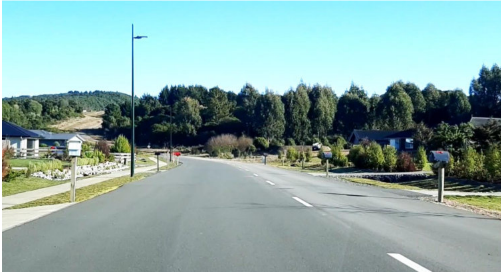
Figure 10 Cross Section of Kahikatea Drive east of its intersections with Oakdale Drive
