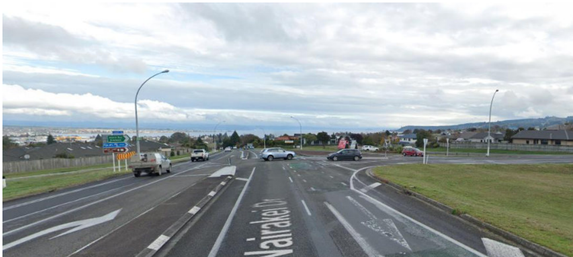
Figure 26: Wairakei Road / Pohipi Road Intersection (Source: Google Streetview looking south)
