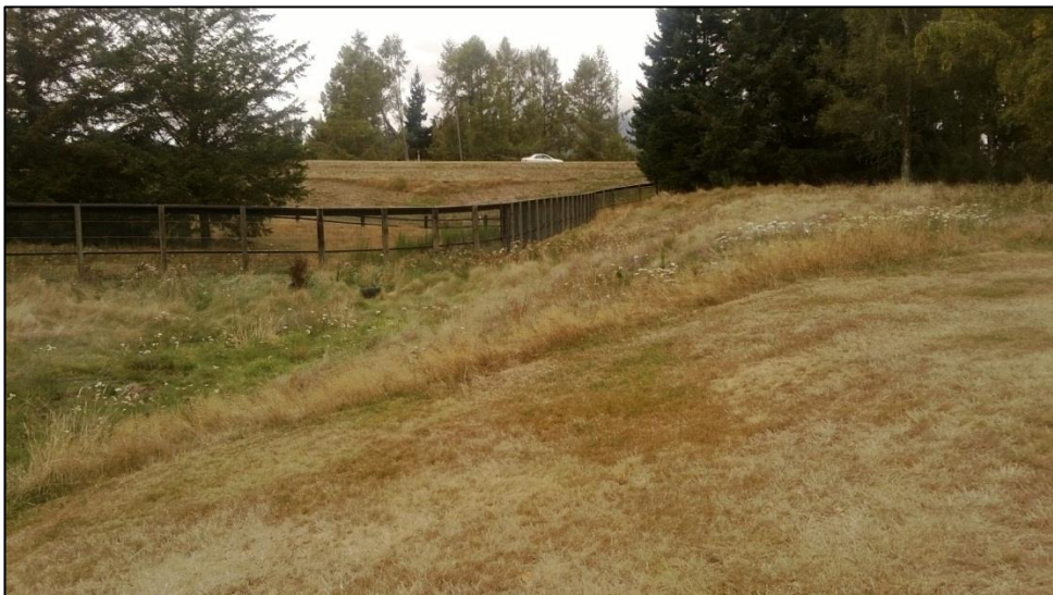
FIGURE 5: VIEW OF STORMWATER DRAINAGE CHANNEL/SWALE ON EASTERN BOUNDARY THE FIRST TEE AT WAIRAKEI INTERNATIONAL GOLF COURSE
