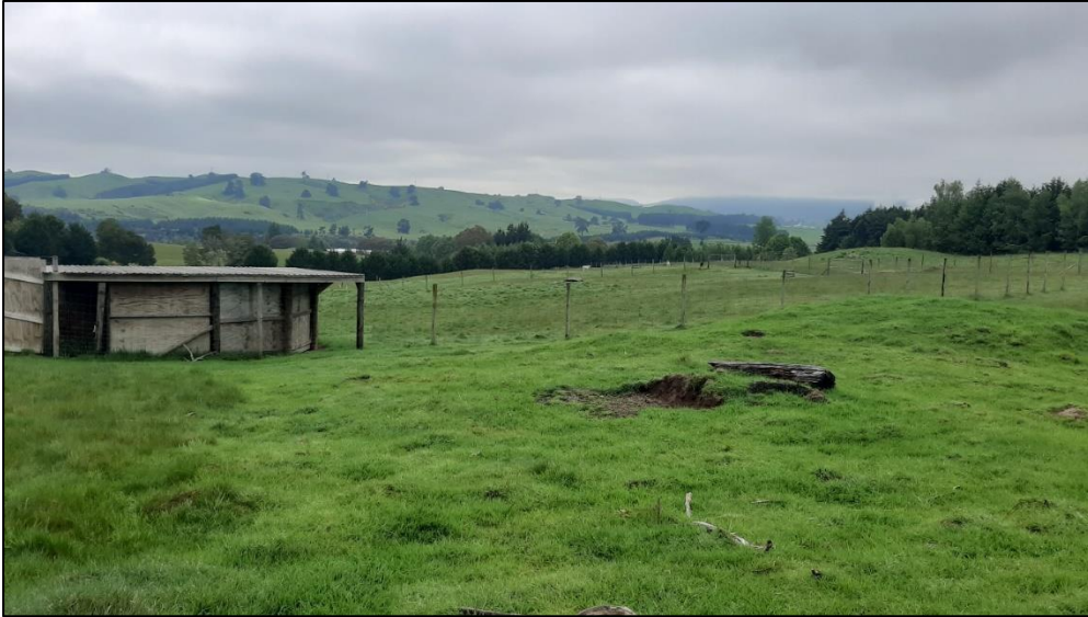
PHOTO 2. RUBBLE REMAINS FROM FORMER BUILDING STRUCTURES
