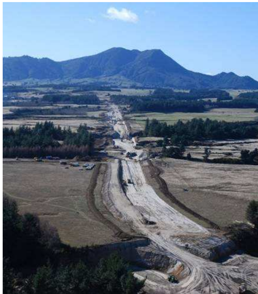
East Taupō Arterial under construction
