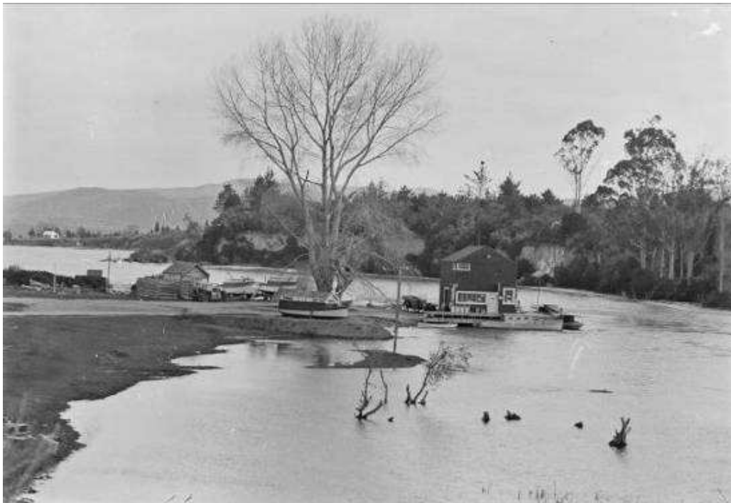
Illustration 32: 1928, wharf and small jetty on Taupo Landing Reserve, the double storey corrugated iron shipping office was replaced in 1937 by a single storey wooden building from Napier and that building was later incorporated into subsequent alterations to the wharf. Alexander Turnbull Library, Reference No. APG-1913-1/2-G.
