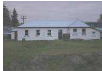
Illustration 9: Old Taupo Courthouse, built 1881, altered 1887, now the Kohanga Reo, AM 2008.
