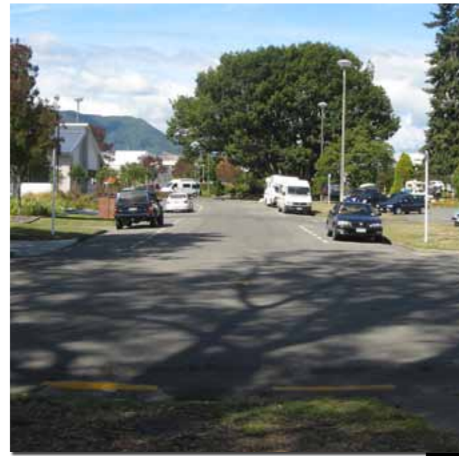
Dead end streets such as Story Place can be reconnected into the network. ✗
