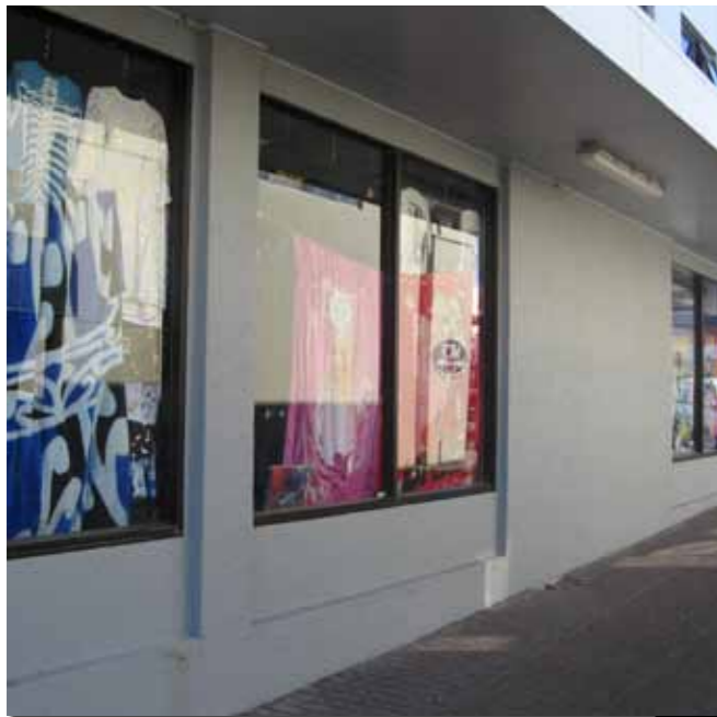
Adjoining activities should relate to the laneway rather than blocking it out. ❌
