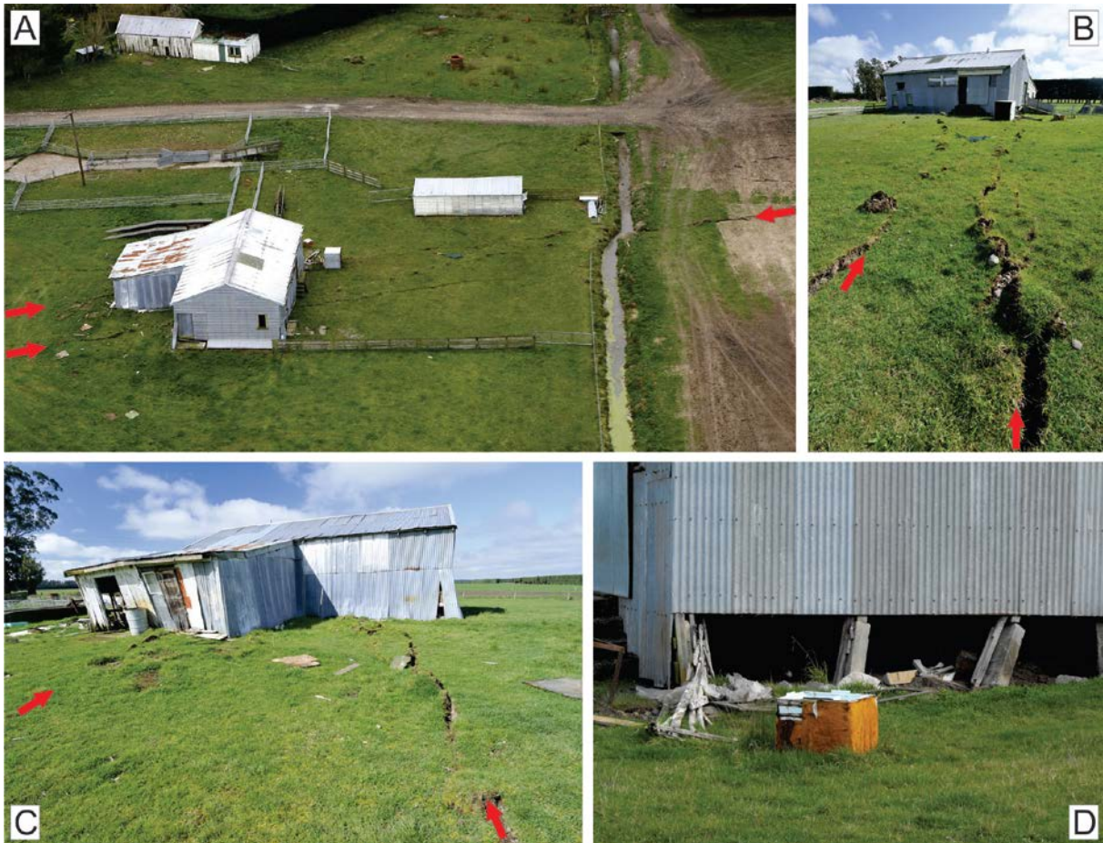
Figure A2.11 Kivers Road woolshed and Greendale Fault surface rupture; see Figures A2.7 and A2.8 for location. Red arrows denote location of discrete surface fault rupture. (A) Aerial view looking northeast – note dextral offset of irrigation channel in right-hand side of photograph. Photo by Richard Cosgrove. (B) View looking west. Photo by Dougal Townsend. (C) View looking east. Photo by Dougal Townsend. (D) View looking southwest showing detail of shallow-seated concrete piles. Photo by Russ Van Dissen.
