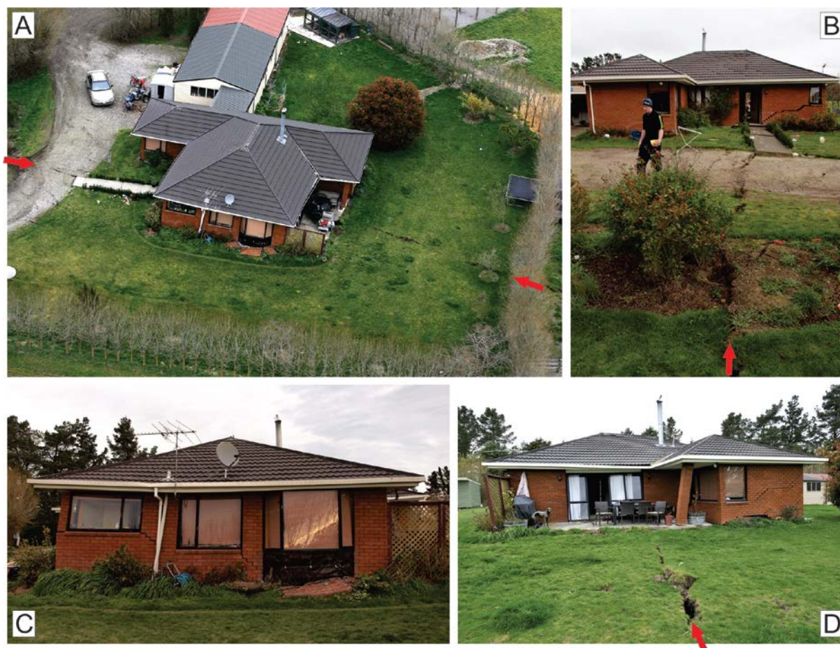
Figure A2.10 Telegraph Road house and Greendale Fault surface rupture; see Figures A2.7 and A2.8 for location. Red arrows denote location of discrete surface fault rupture. (A) Aerial view looking south. Photo by Richard Cosgrove. (B) View looking west-northwest. Photo by Hayden Mackenzie. (C) View looking south-southwest. Photo by Hayden Mackenzie. (D) View looking east-southeast. Photo by Dougal Townsend.
